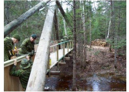
Working on the Suspension Bridge.
